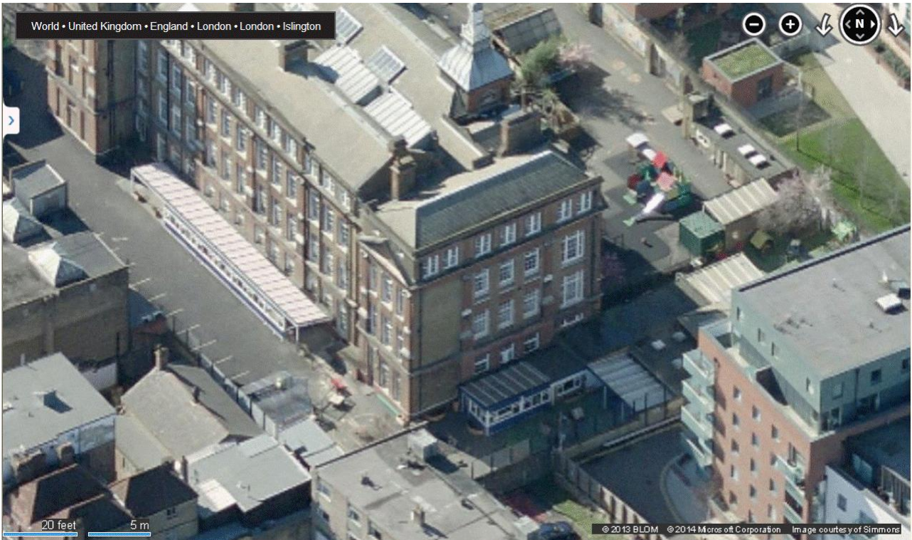
Image 1: The school and site, north east elevation
